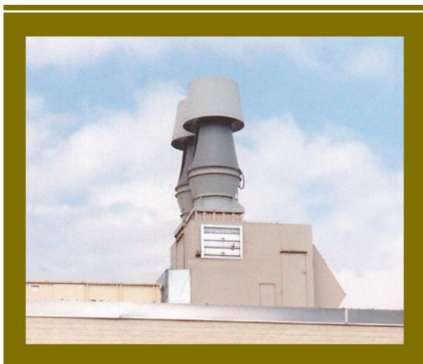
Figure 5: Two mixed-flow impeller systems mounted on top of a heat-recovery system.
