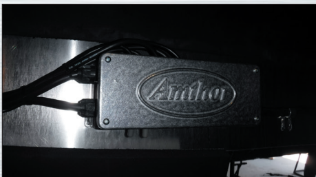
Small watertight casted aluminum electrical box installed in the rear canopy, bucket box, or side cabinet.
