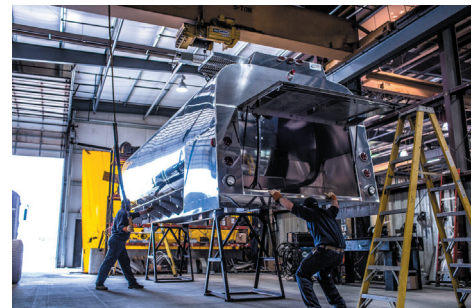
Mounting - this stage is where the tank is installed on the truck chassis of your choice. Piping and equipment is installed in this stage.
