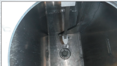
Standard calibration markers installed on top of the tank with a disc that is set to read the proper gallon use in the tank.
