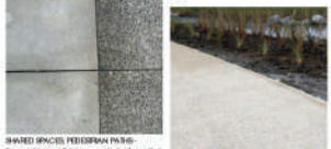
PAVED AREAS 600x400x40mm brick pavers (paved path) and 100mm wide saw-cut exposed aggregate concrete (edge detail)
