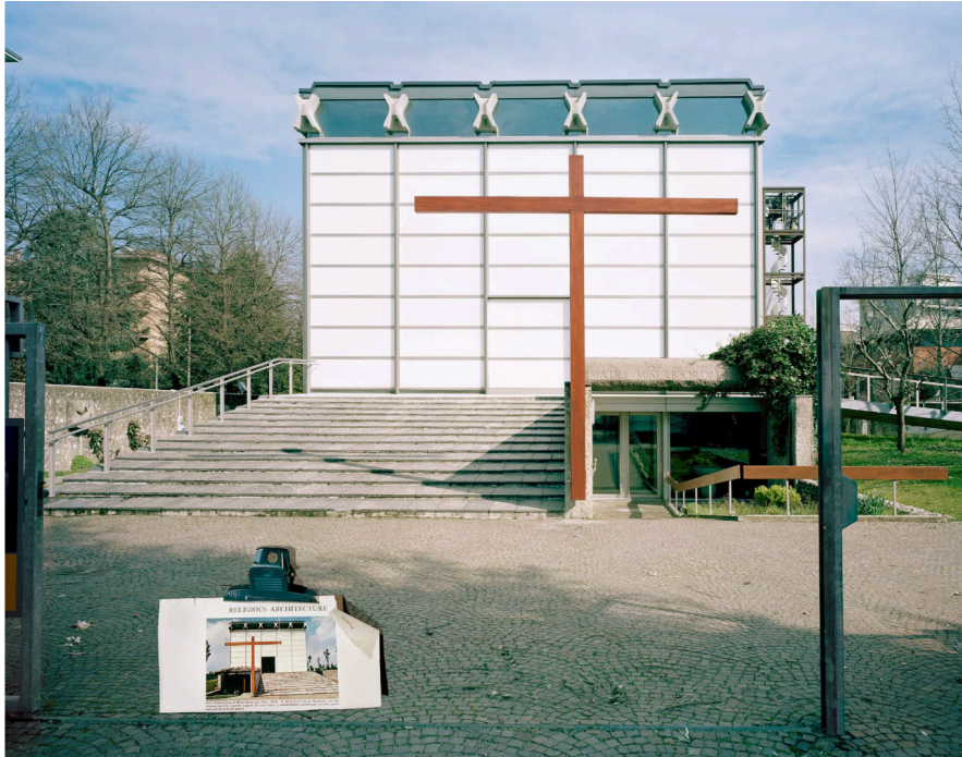
"Nostra Signora della Misericordia Church, Italy (In Progress)," 2023.
