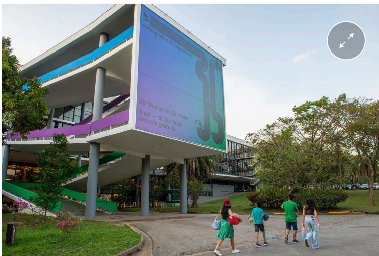
The Cicillo Matarazzo Pavilion, by Oscar Niemeyer, where the São Paulo Biennial is taking place. LEVI FANAN
