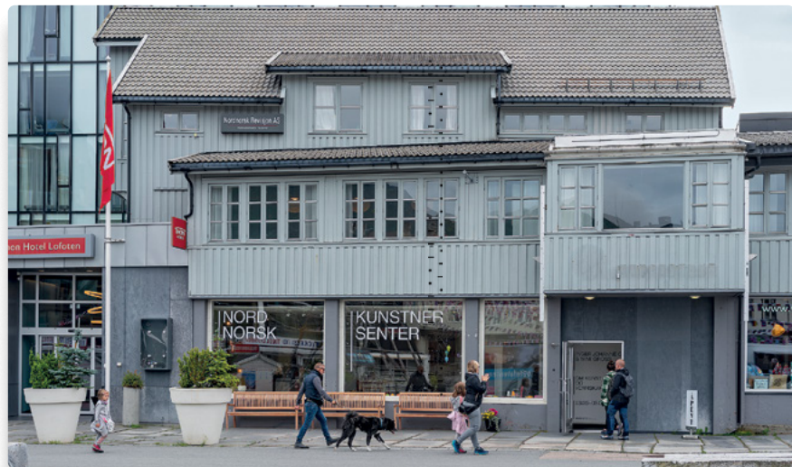
The North Norwegian Art Centre located at the main square in Svolvær. Photo: Kjell Ove Storvik
