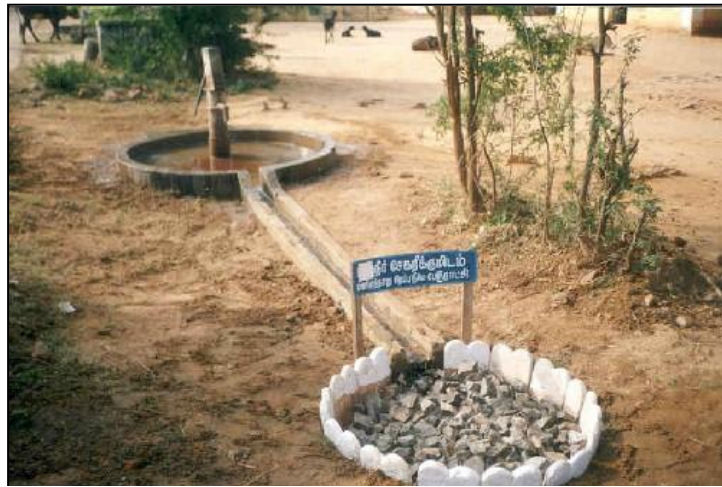
Unused water re-circulated into aquifer (Rain Water Harvesting, DTP, 2006)
