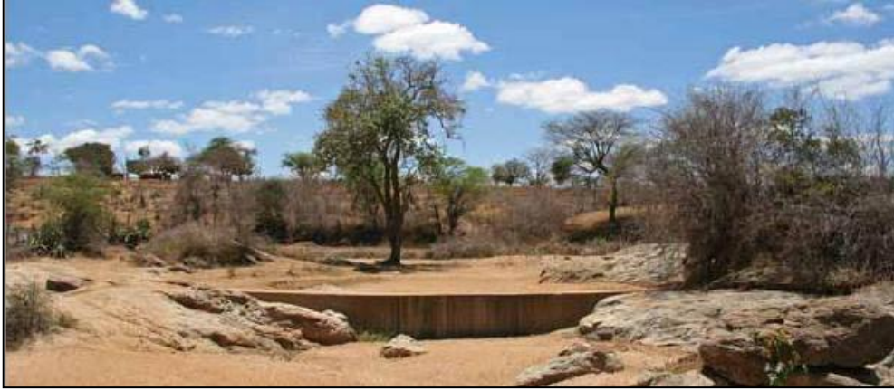
Sand dam in Kitui district of Kenya: (New Scientist Nov 2006)
