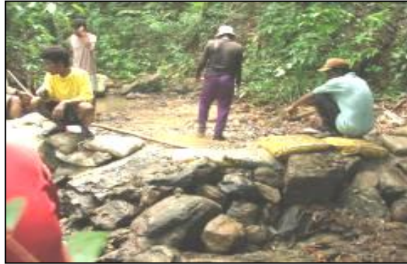
Construction of a check dam ( www.undop.or.th , n.d)
