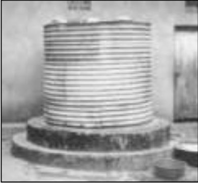
Corrugated steel tank in Uganda (DTU, 2002)
