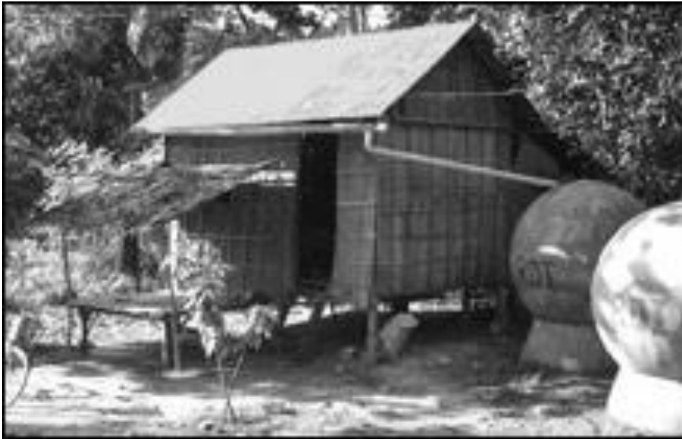
Cambodian household with a sheet metal roof used for rainwater harvesting ( Resource Development International Cambodia, n.d. )
