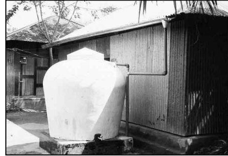
Mortar tank in Bangladesh (Rainwater Toolkit, 2005)
