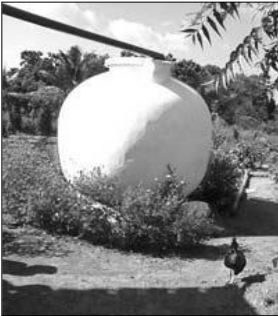
Spherical pumpkin tank design in Sri Lanka (ITDG South Asia, n.d.)
