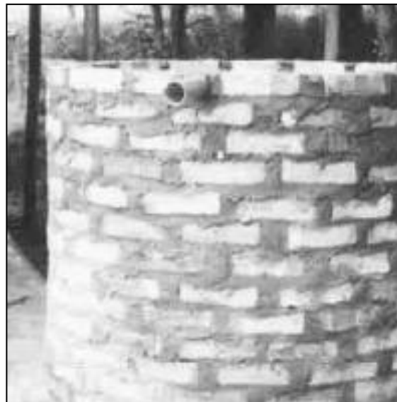
Figure: Brick jar under construction in Uganda
