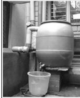
Plastic tank in India (Bangalore Rainwater Club)
