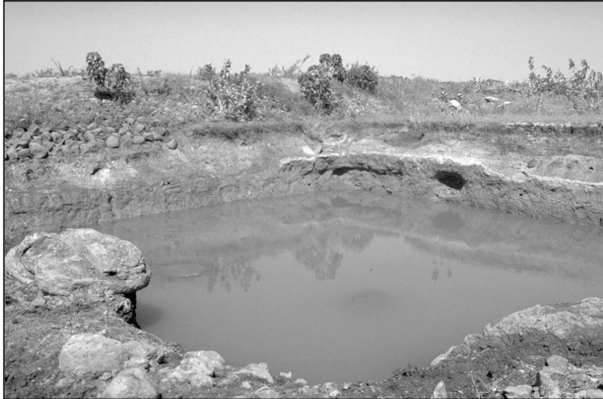
Figure: Constructed oorani in Mayarundi for water harvesting. The last rainfall was received about 45 days previous.
