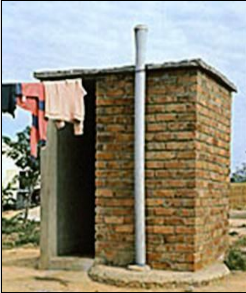
Ventilated Improved Latrine (VIP)
