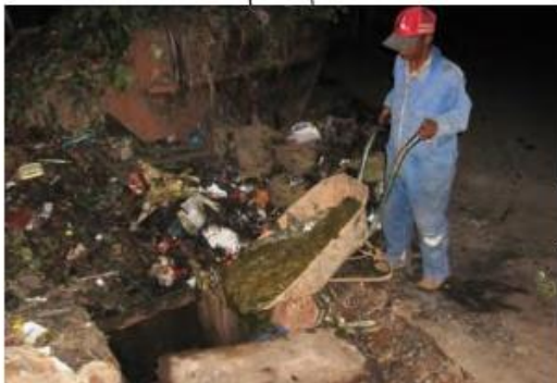
Discharging in a manhole or burying in a trench
