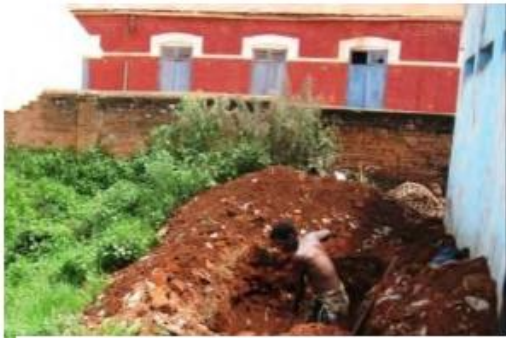
Digging the trench for burying sludge
