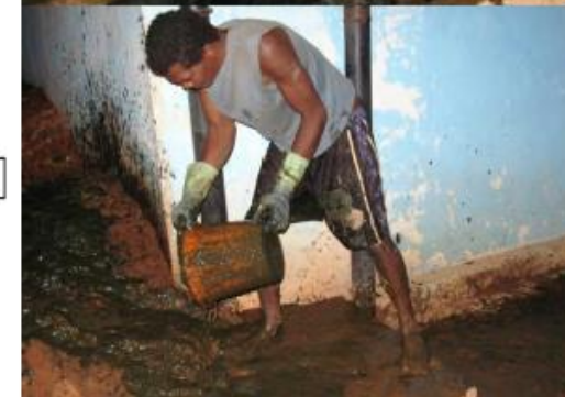
Removing the sludge
