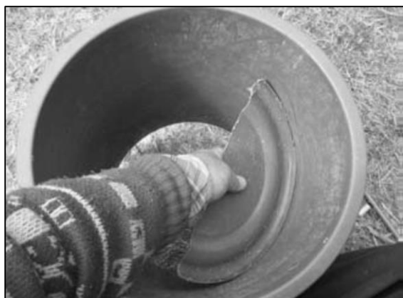
Step 3. Connect one half of the base half way up the bucket using wire. The base should be at an angle so that it will collect urine.
