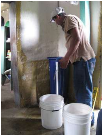
Plastic filter installation
