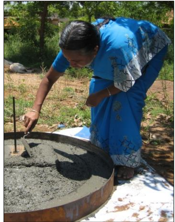
CAWST training on how to build a latrine slab, India
