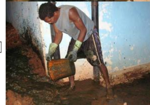
Removing the sludge
