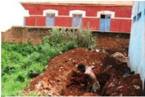
Digging the trench for burying sludge
