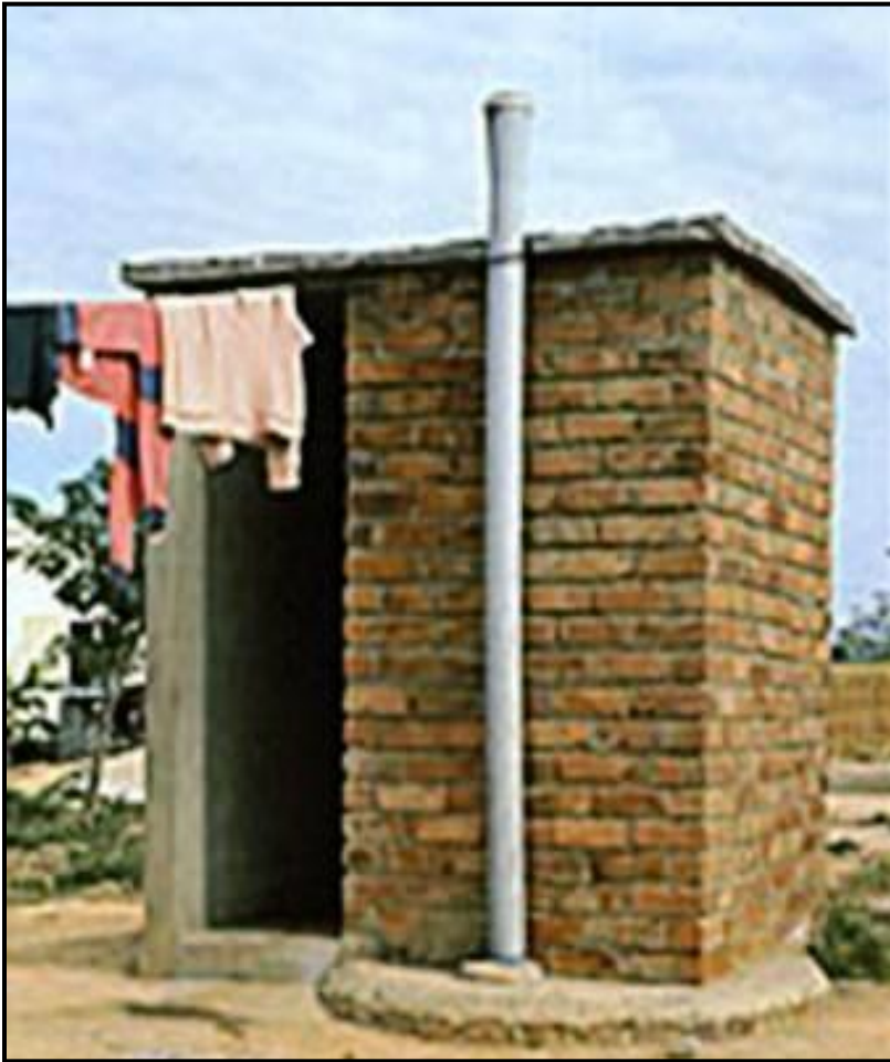
Ventilated Improved Latrine (VIP)
