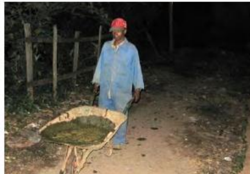
Transferring the sludge
