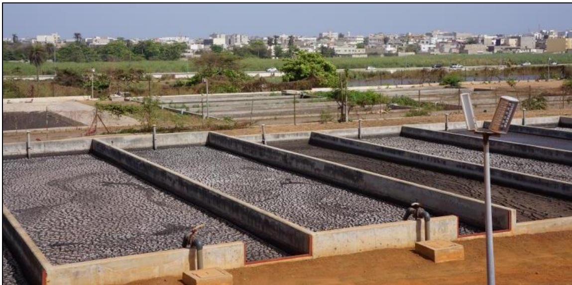
Unplanted drying beds at a faecal sludge treatment facility in Dakar, Senegal (Credit: Eawag-Sandec)
