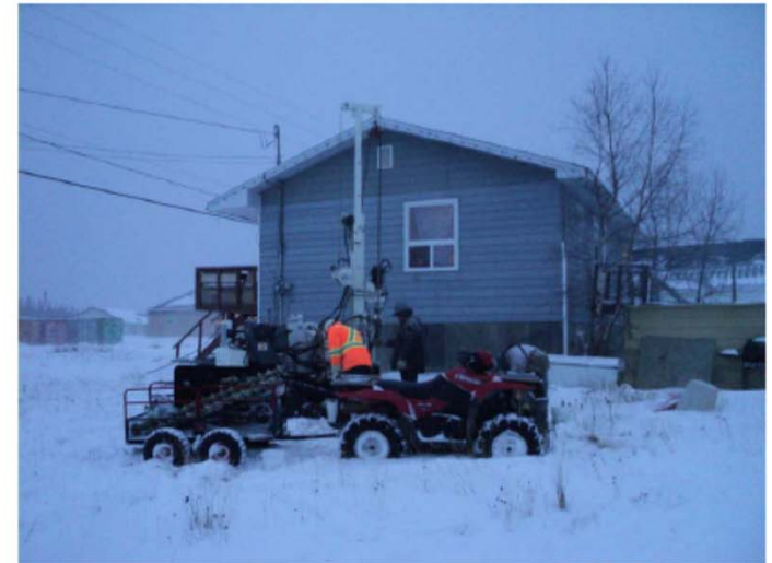
Photo 4: Photo of drilling monitoring well MW205.
