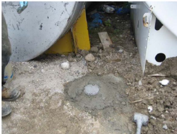
Photo 2: Photo of monitoring well MW102 installed between the bases of two ASTs.
