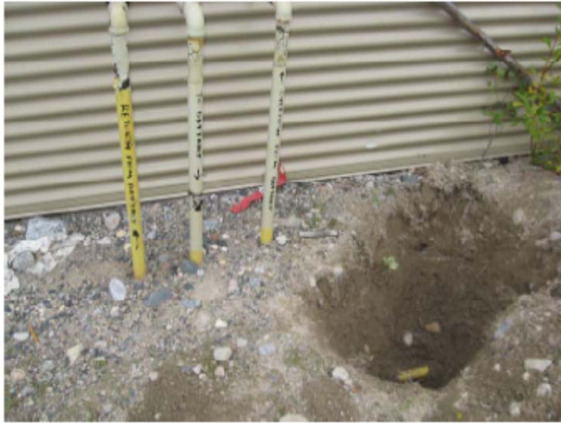
Photo 4: Photo of borehole K-FL-1 installed along fuel distribution line extending from the bulk fuel storage facility to the Education Centre.
