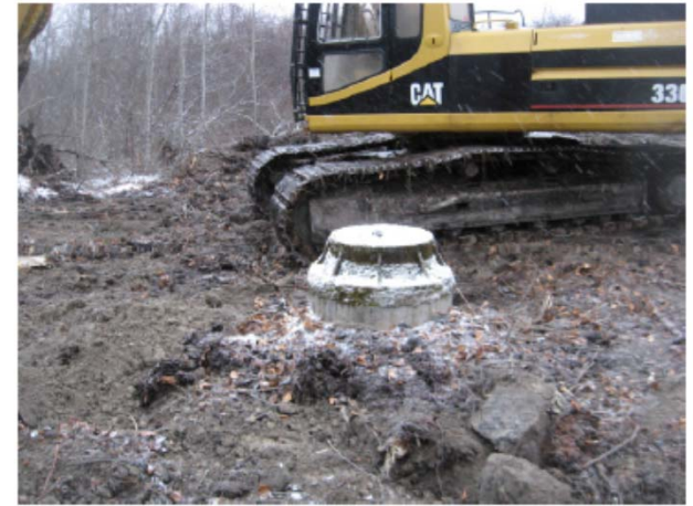
Photo 4: Photo of manhole located between former building and shore of Attawapiskat Lake. Note that test pit TP110 was advanced along discharge pipe extending from former sewage plant to manhole.
