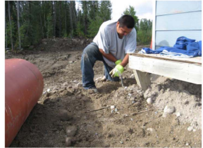
Photo 3: Photo of hand-auguring activities at Building 6. Note that the AST was temporarily removed from the wooden platform to facilitate installation of new weeping tiles around building.
