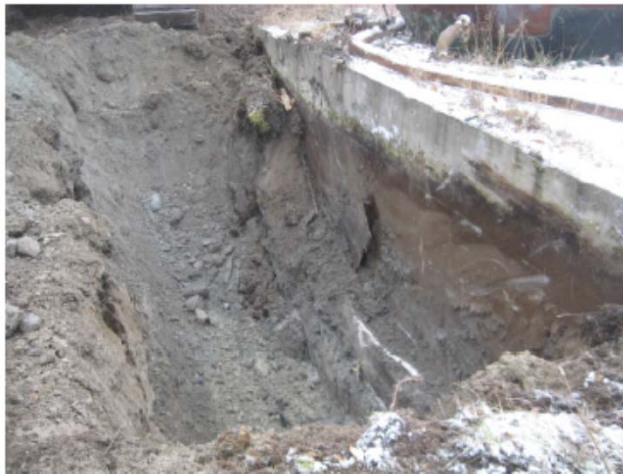
Photo 3: Photo of investigation adjacent to concrete foundation associated with former sewage treatment plant building.
