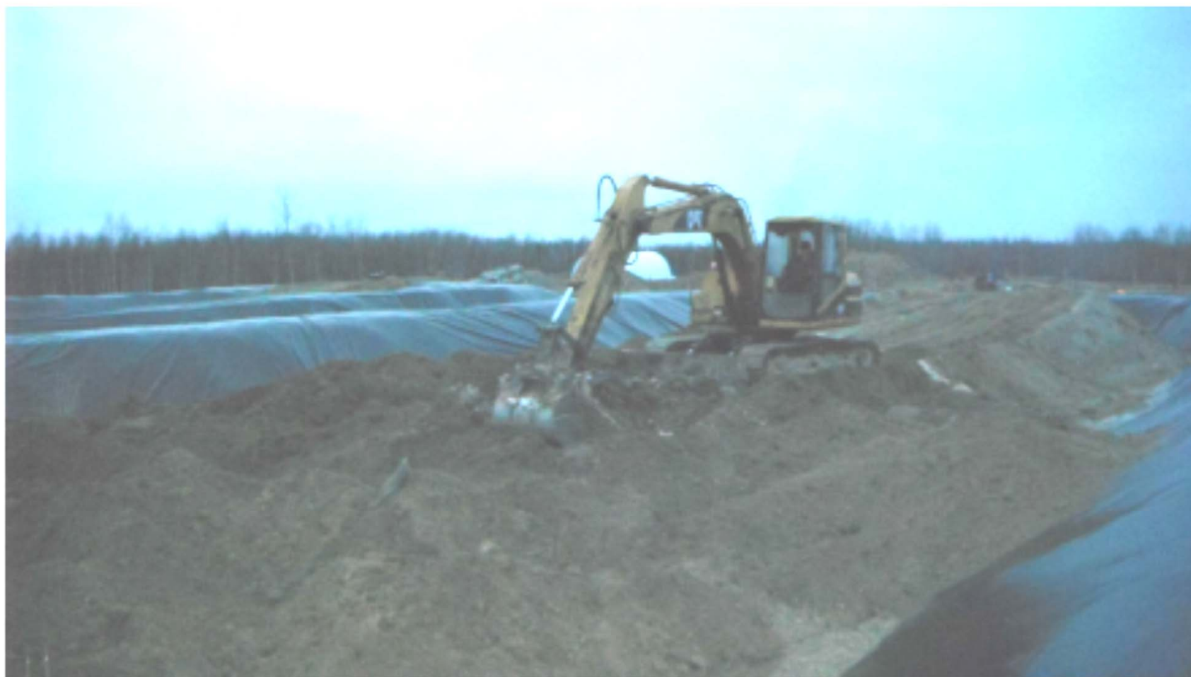
Photo 3: Photo of soil tilling activities completed at Cell 2 during the 2014 Treatment Season.
