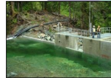
Run-of-river hydro at Canoe Creek, Tla-o-qui-aht First Nation, BC
