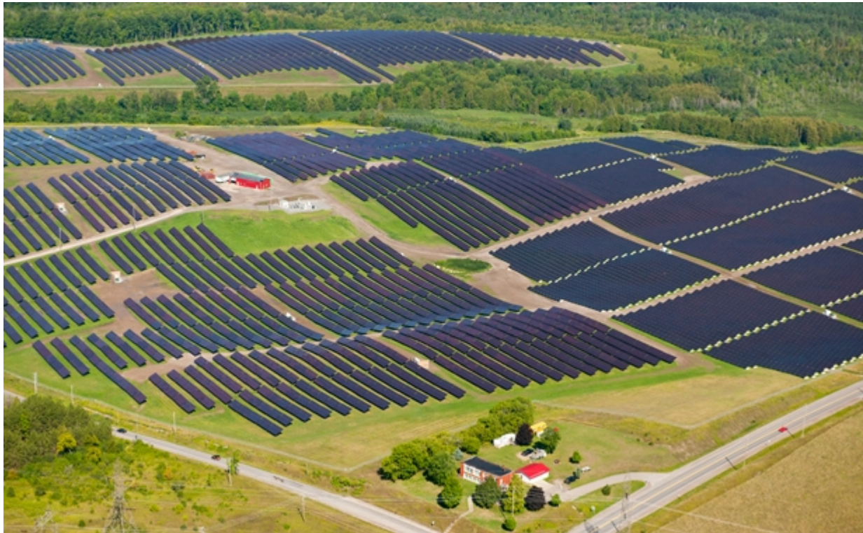
10MW Solar Farm
