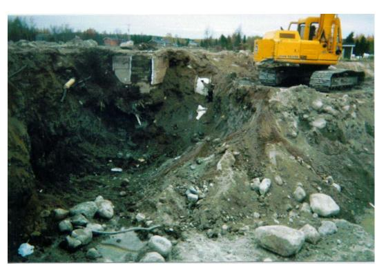
Contaminated soils are either relocated and treated in a contained facility, or left in place and treated in ground with the use of additives.
